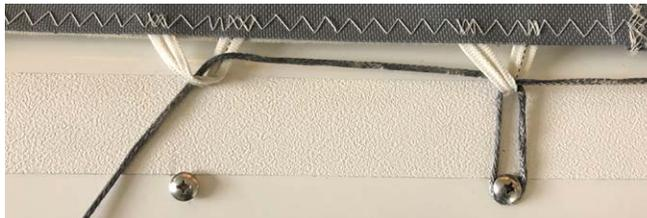
12. Loop around the bolt and continue **underneath** the line.
