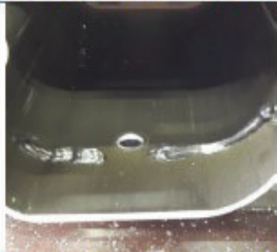
C. Clean the surface and put sikaflex or puraflex in front of the hole for the beambolt.
